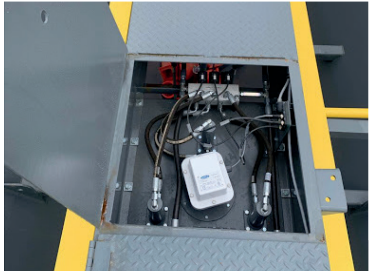
07/ HINGED WALKWAY PLATES
